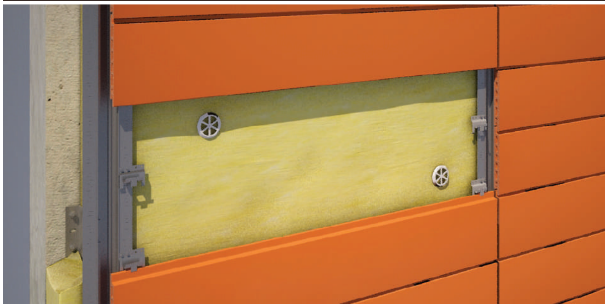
Installation on metal framework
